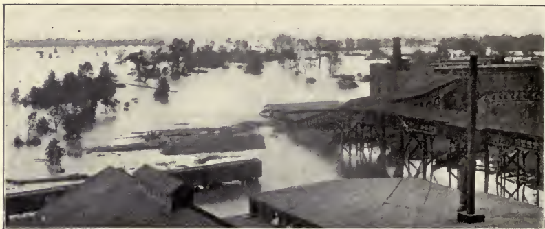
Venice and East Madison Streets where buildings were completely submerged and swept away
